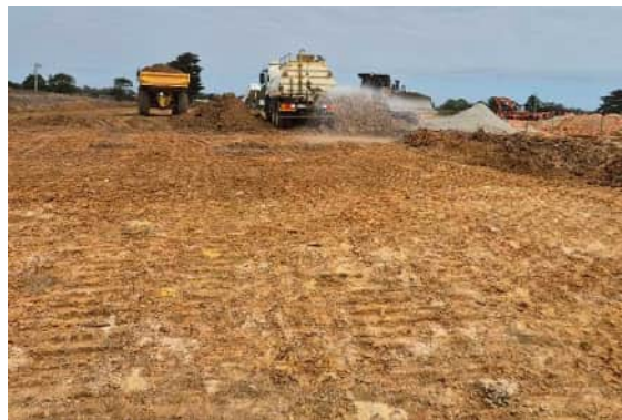
Photograph 8: Water cart conditioning clay
