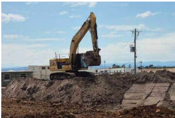
Photograph 7: Excavator moving earth
