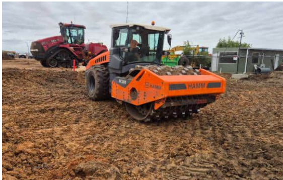
Photograph 5: Vibrating pad foot roller preparing fill
