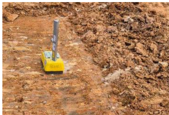
Photo 10: Field density/moisture test
