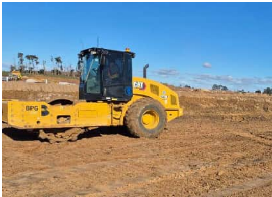
Photograph 5: Vibrating pad foot roller used during fill construction.
