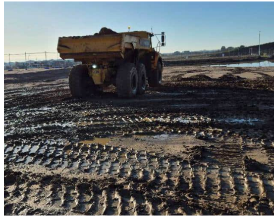
Photograph 4: Subgrade assessment using loaded dump truck.
