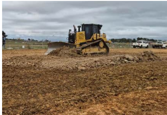
Photograph 6: D6 Dozer spreading clay.
