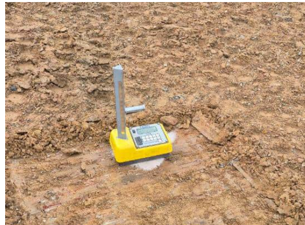
Photo 10: Field density/moisture test
