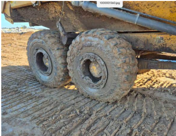
Photograph 3: Subgrade assessed with dump truck.
