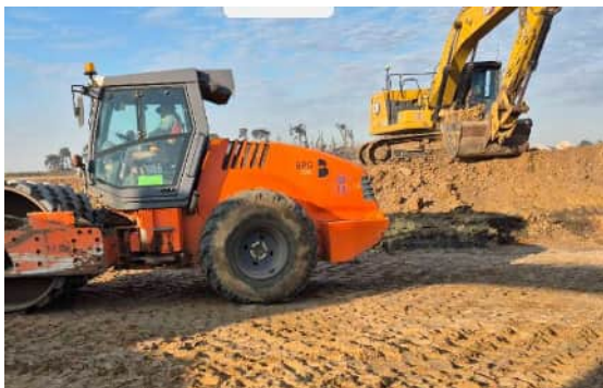
Photograph 7: Excavator and vibrating pad foot roller used during construction.
