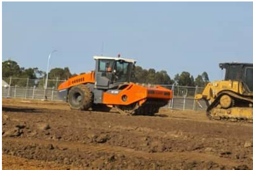
Photograph 5: Pad foot used during fill construction
