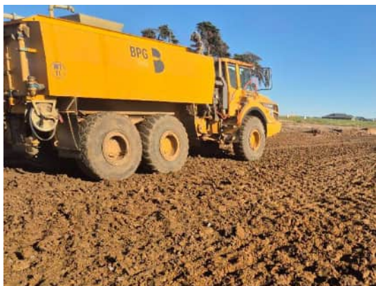
Photograph 3: Subgrade assessed with water truck
