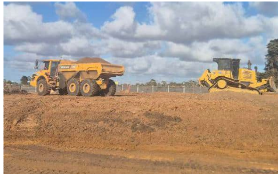
Photograph 6: Import of materials used during fill construction
