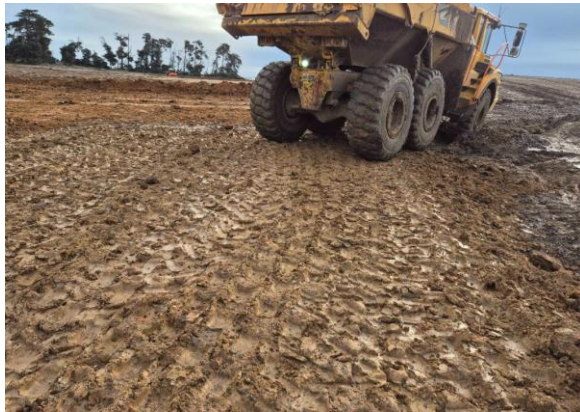
Photograph 3: Subgrade assessed with dump truck
