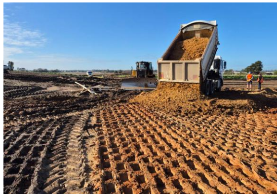
Photograph 8: Dozer spreading material during fill construction
