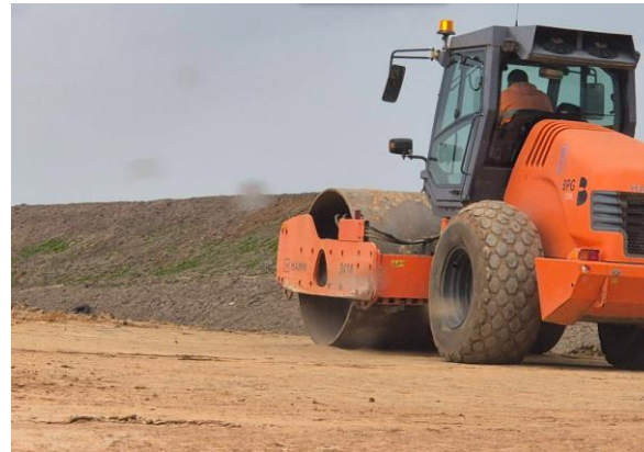
Photograph 4: Subgrade assessment using smooth drum roller
