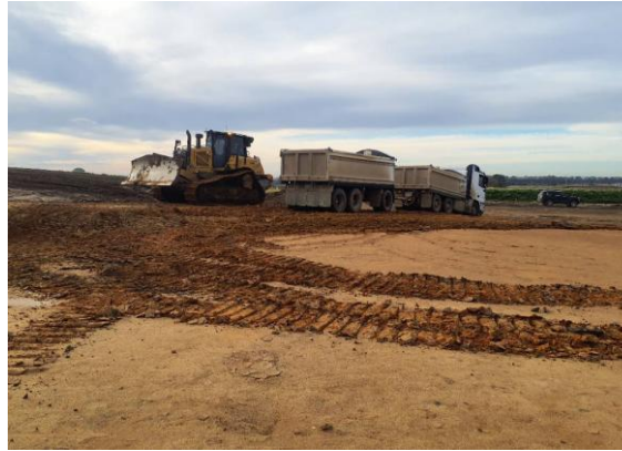
Photograph 6: Import of materials used during fill construction
