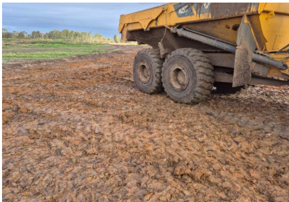
Photograph 7: Moxxy placing clay during fill construction
