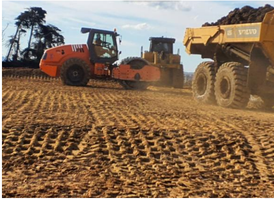
Photograph 5: Pad foot used during fill construction
