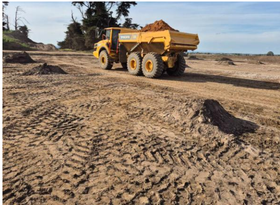
Photograph 3: Subgrade assessed with dump truck
