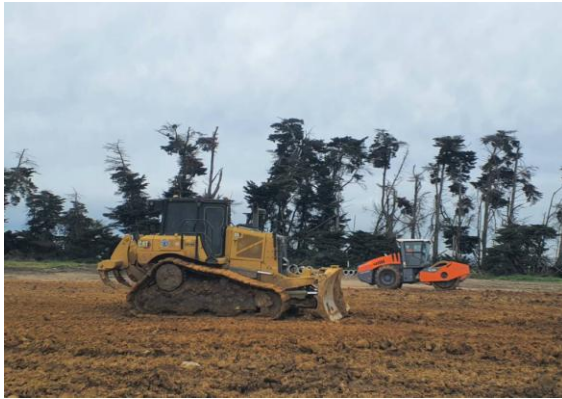
Photograph 5: Dozer used during fill construction
