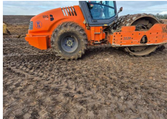
Photograph 4: Subgrade assessment using pad foot roller
