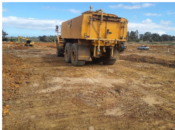
Photograph 4: Subgrade assessment using loaded water cart
