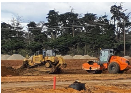
Photograph 6: Pad foot and Dozer used during fill construction
