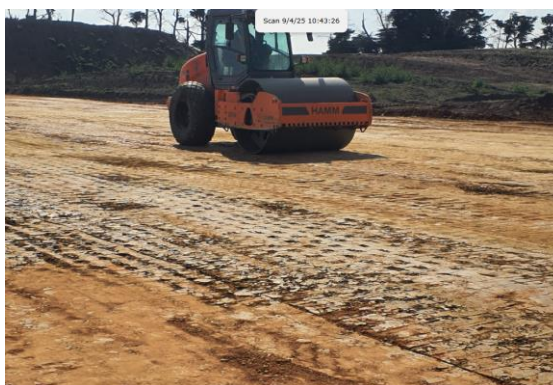
Photograph 8: Smooth drum roller used during fill
