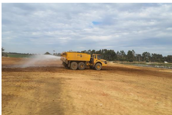
Photograph 7: Water cart during fill construction
