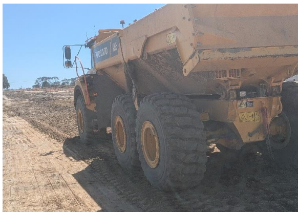
Photograph 3: Subgrade assessed with dump truck
