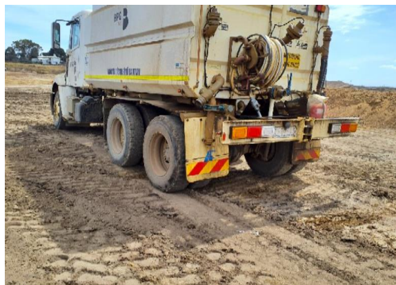
Photograph 4: Subgrade assessment using loaded water cart
