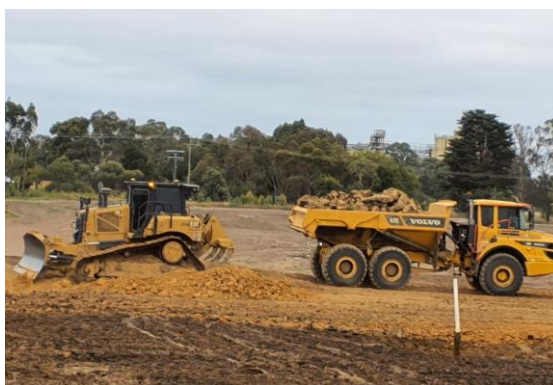
Photograph 8: Moxxy trucks used during fill construction
