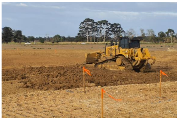
Photograph 5: Dozer used during fill construction
