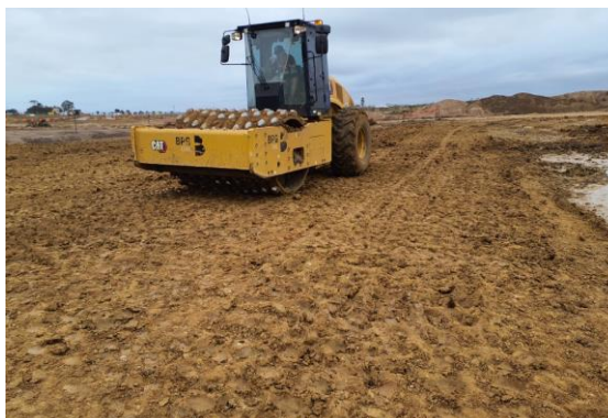
Photograph 6: Pad foot used during fill construction
