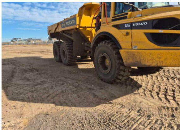
Photograph 3: Subgrade assessed with dump truck
