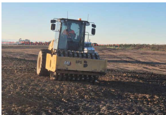
Photograph 7: Vibrating compactor used during fill construction
