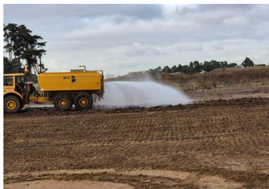
Photograph 8: Water Cart used during fill construction
