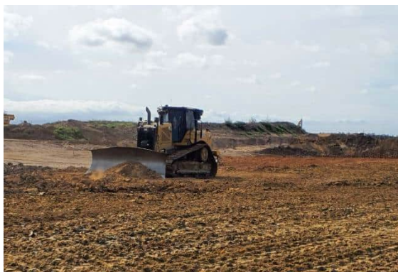
Photograph 5: Dozer used during fill construction
