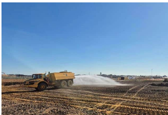
Photograph 7: Water cart during fill construction
