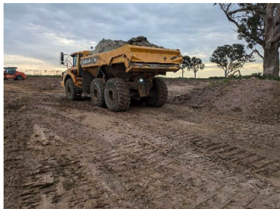
Photograph 4: Subgrade assessment using loaded dump truck
