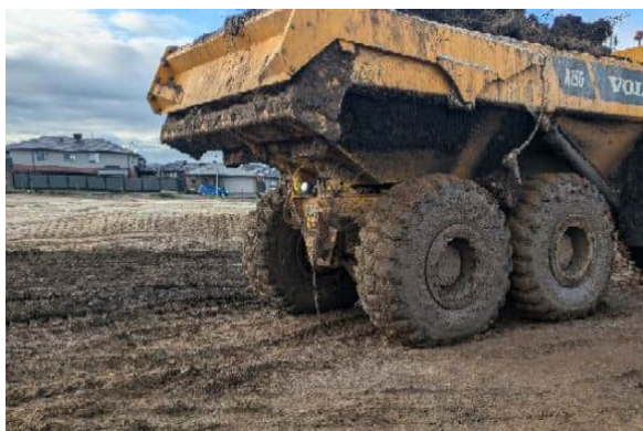
Photograph 3: Subgrade assessed with dump truck
