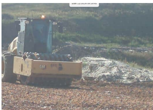
Photograph 7: Compactor used during fill construction
