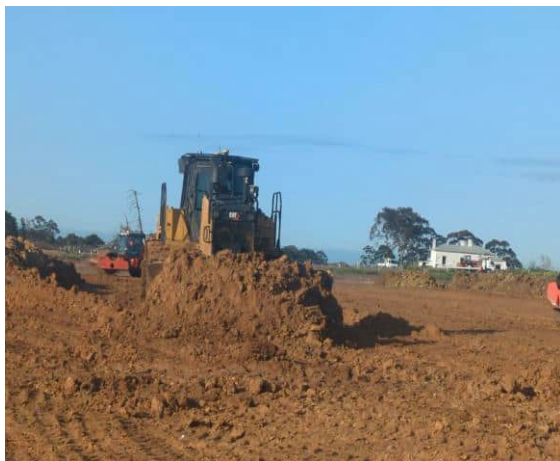
Photograph 5: Dozer used during fill construction
