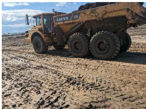
Photograph 4: Subgrade assessment using loaded dump truck
