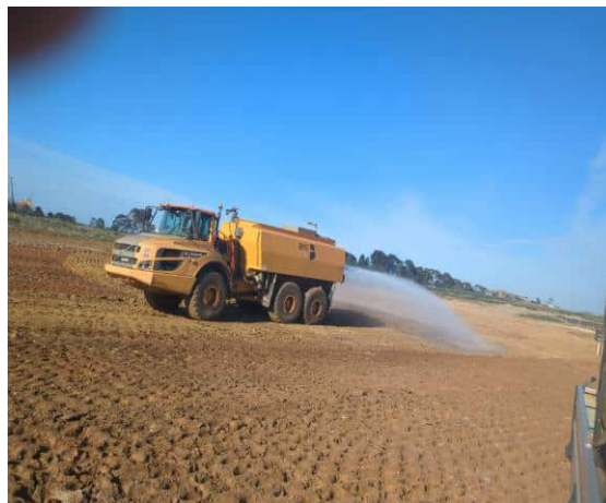
Photograph 6: Water cart used during fill construction
