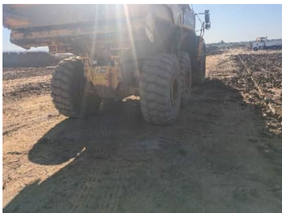
Photograph 3: Subgrade assessed with dump truck
