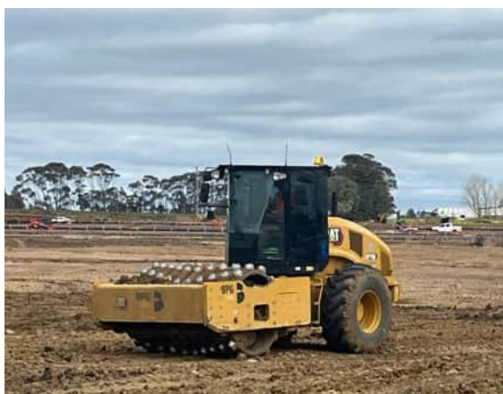
Photograph 7: Compactor used during fill construction
