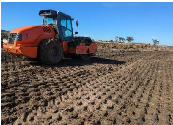
Photograph 3: Subgrade assessed with pad foot roller
