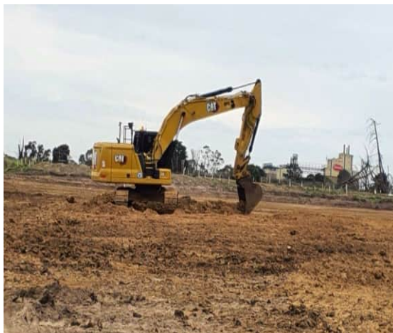
Photograph 6: Excavator used during fill construction
