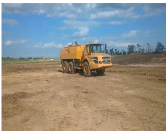
Photograph 8: Water cart used during fill construction
