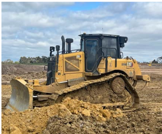
Photograph 5: Dozer used during fill construction
