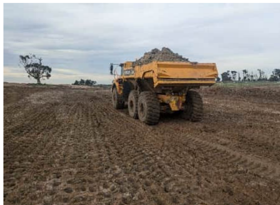
Photograph 4: Subgrade assessment using loaded dump truck
