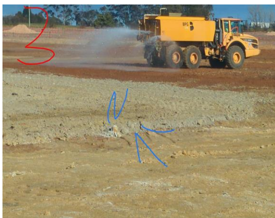
Photograph 8: Water cart used during fill construction
