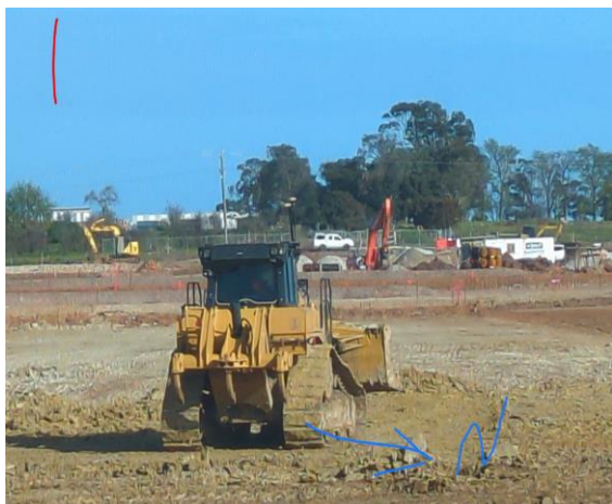
Photograph 5: Dozer used during fill construction
