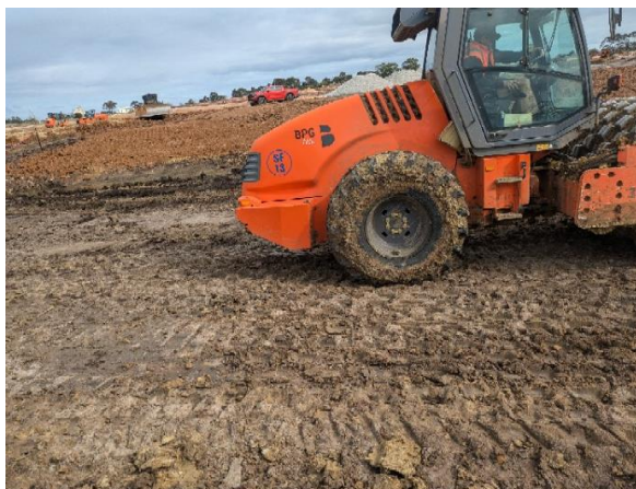
Photograph 3: Subgrade assessed with Pad foot roller
