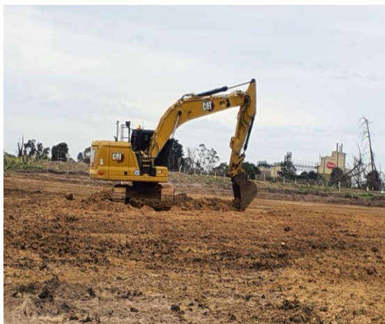
Photograph 6: Excavator used during fill construction
