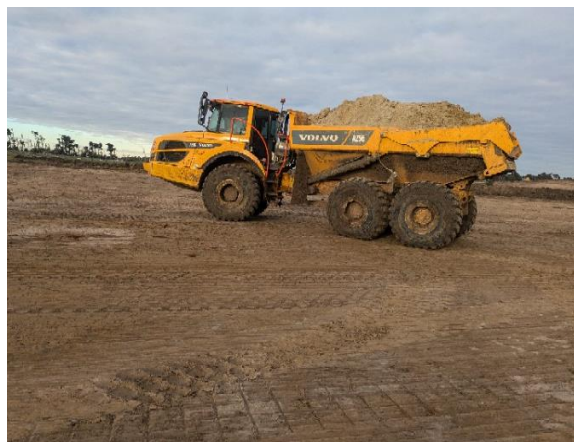
Photograph 4: Subgrade assessment using loaded Dump Truck
