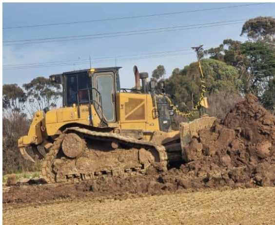
Photograph 5: Dozer used during fill construction
