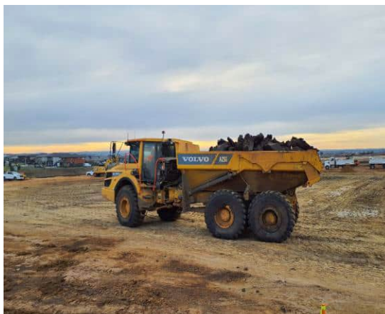
Photograph 8: Moxxy trucks used during fill construction
