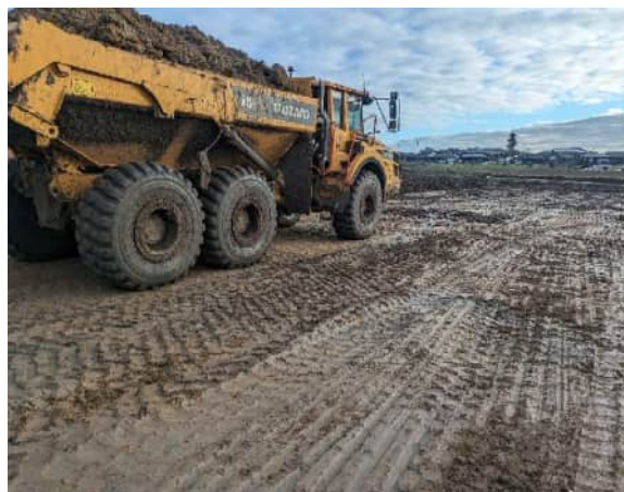
Photograph 4: Subgrade assessment using loaded dump truck
