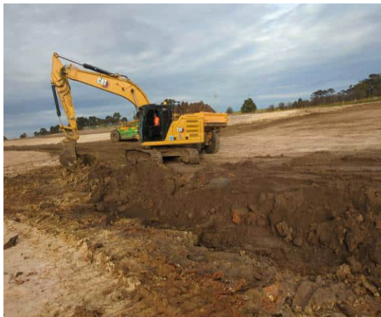
Photograph 6: Excavator used during fill construction
