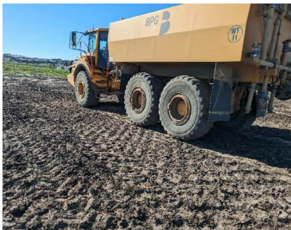
Photograph 3: Subgrade assessed with watercart
