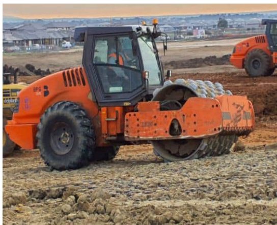
Photograph 7: Compactor used during fill construction
