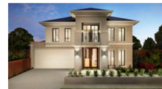
Carlisle – Classique • Remove decorative balustrading
