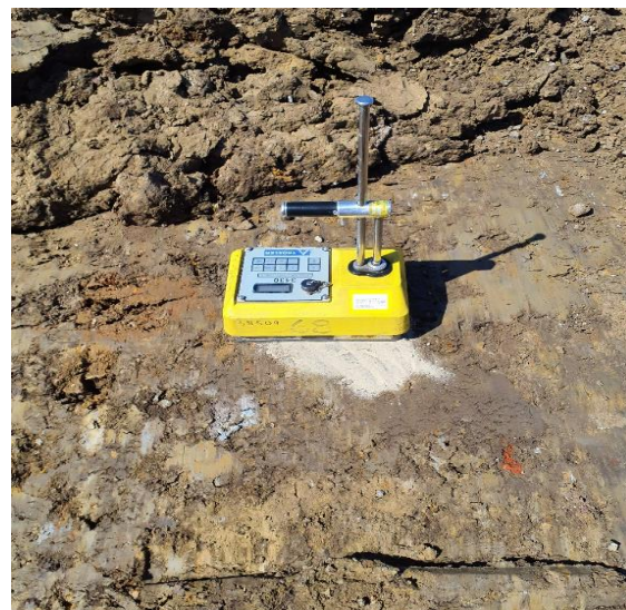
Photo 10: Pad Excavated for Nuclear Density Test
