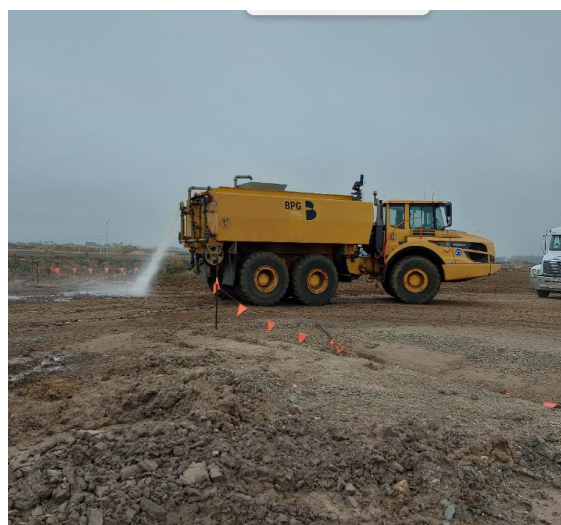
Photo 8: Water cart moisture conditioning
