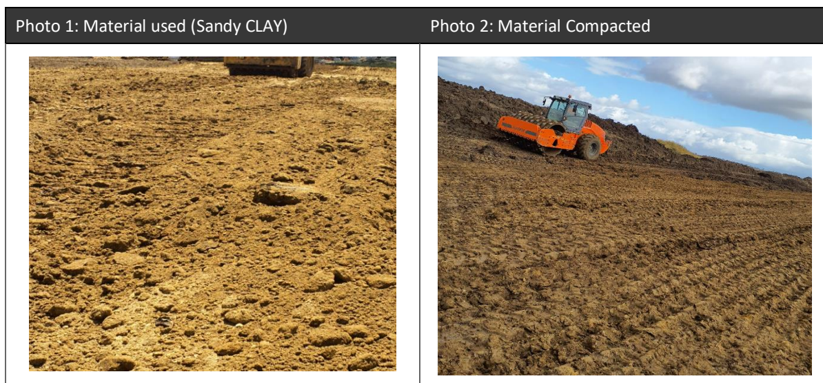
Figure 3.1: Photographs of the material used on site
