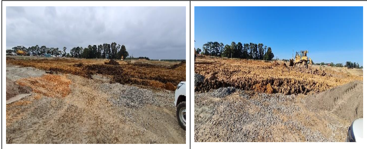
Figure 1. Photograph of the material used on site
