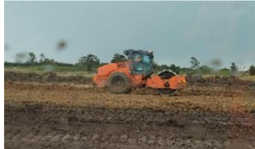
Photograph 2.7.2: Material Compaction
