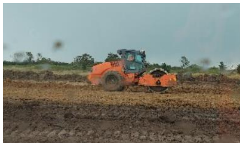
Photograph 2.7.2: Material Compaction
