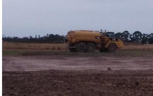
Photograph 2.7.2: Moisture Conditioning material
