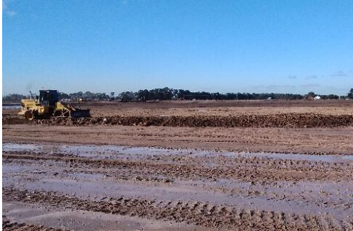
Photograph 2.7.1: Material Compaction and Conditioning
