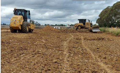
Photograph 2.7.1: Material Compaction
